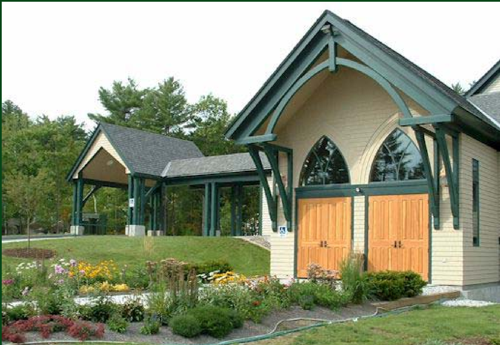
Our Lady of the Mountains Entry and Porte Cochere Painted Douglas Fir Timber with Arched Beams and Deep Chamfers Vermont Timber Works, Inc | vermonttimberworks.com
